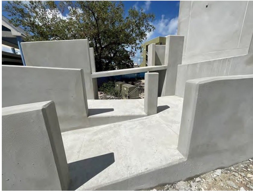
Handicap Ramp after Stucco
