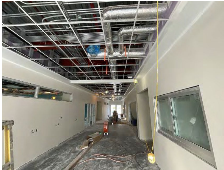
Ceiling Grid Installation
