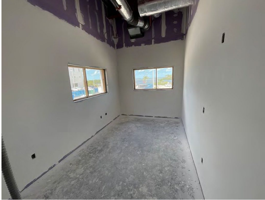
Level 5 Finish with Temp Windows
