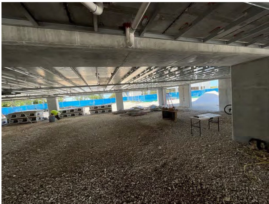
Storage Area Framing
