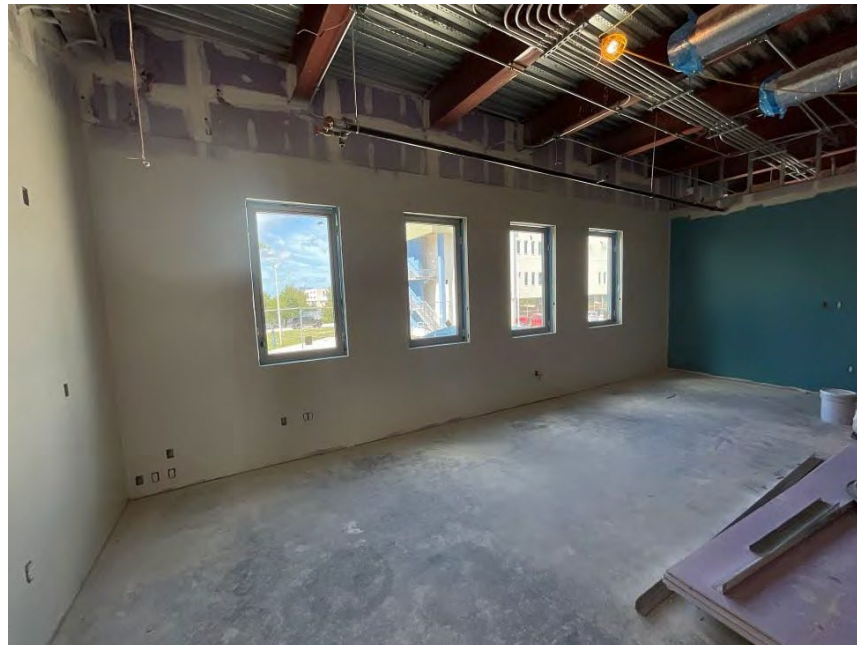
Permanent Window Installation
